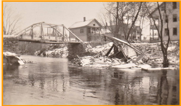
Main Street Temporary Bridge
