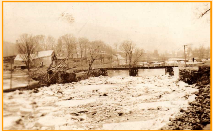
Temporary bridge near Phil French Farm
