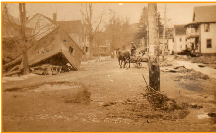
Pearl Street Damage
