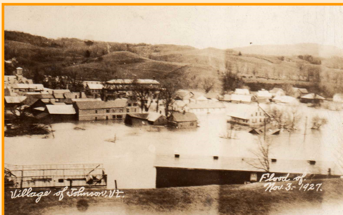
Village Flood Damage
