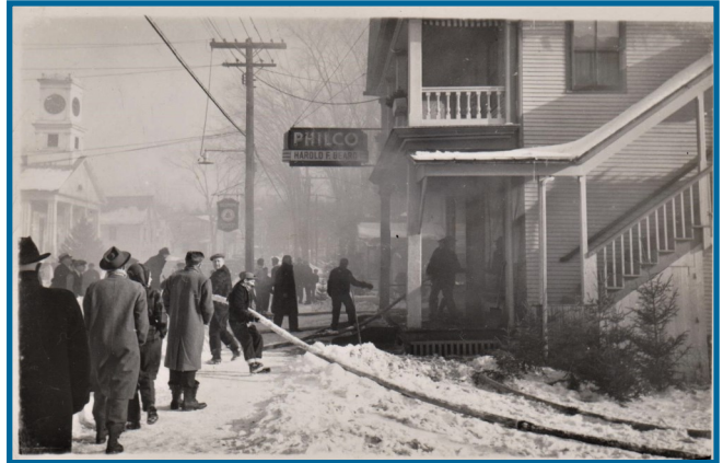
Controlling the fire
