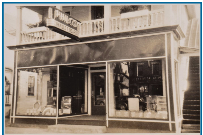
Store front after the windows were added
