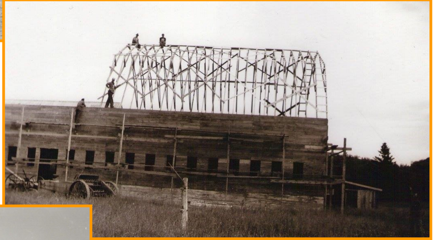
Putting up roof trusses on new barn 1940
