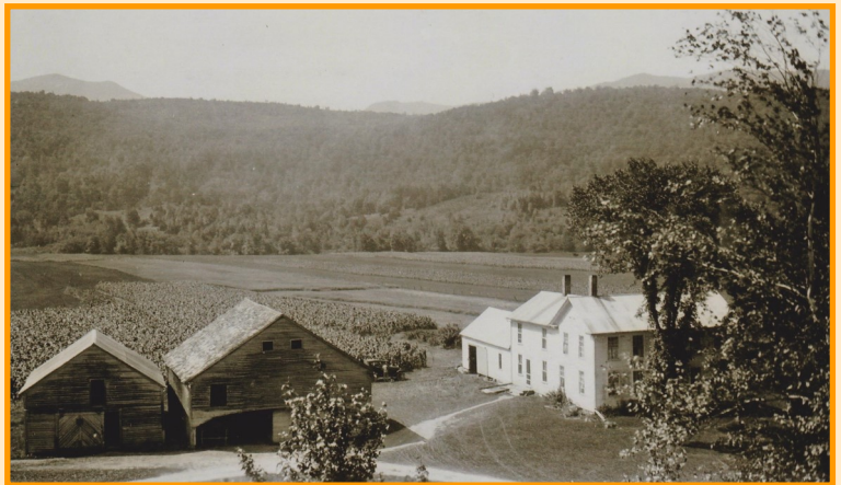
Stiles Ranch 1925--New 2 story addition
