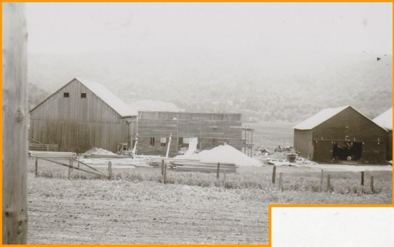
Start of new barn
