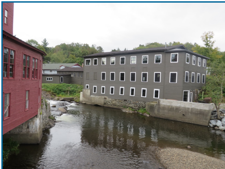
Old Mill on river as it looks today
